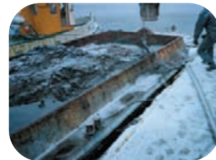
Forurenset muddermasse i leker
